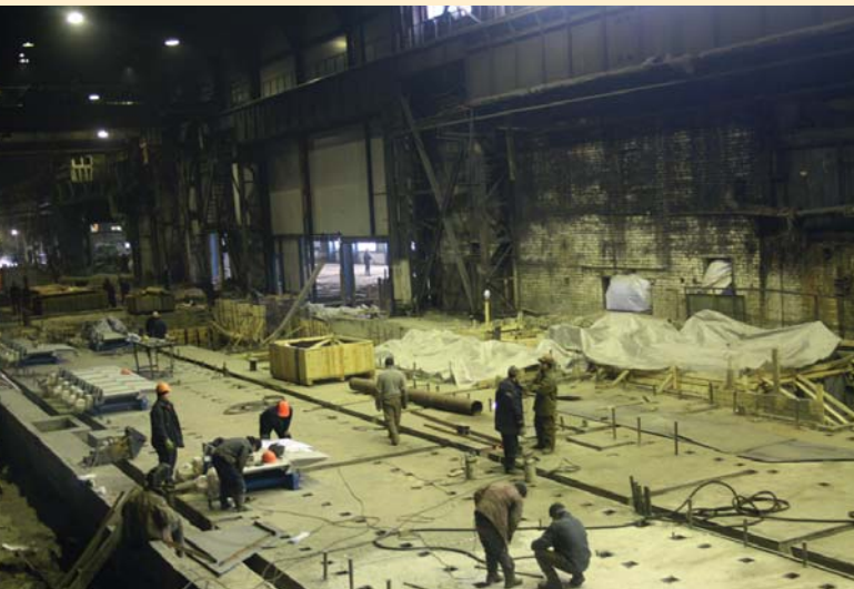
Reconstruction of 500 rolling mill: preparing of basement and mounting of equipment
