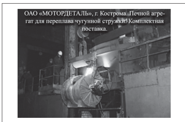
Fig. 8. JSC “Kostromamotordetal” (Kostroma, Russia): the furnace for iron chips melting, full set supply
