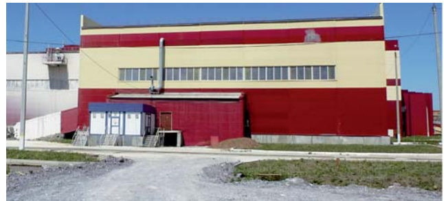
Lime and chemical area
