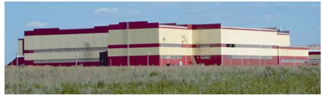
Main building of the processing plant
