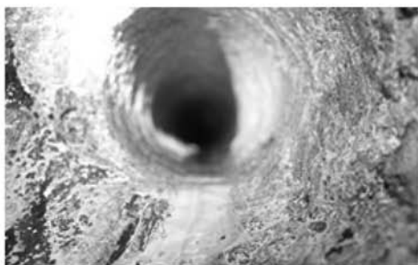
Fig. 1. Horizontal hole no. PS (Ø 105 mm, H = 750 m) with a special white color coating, East site, Tashtagol Mine
