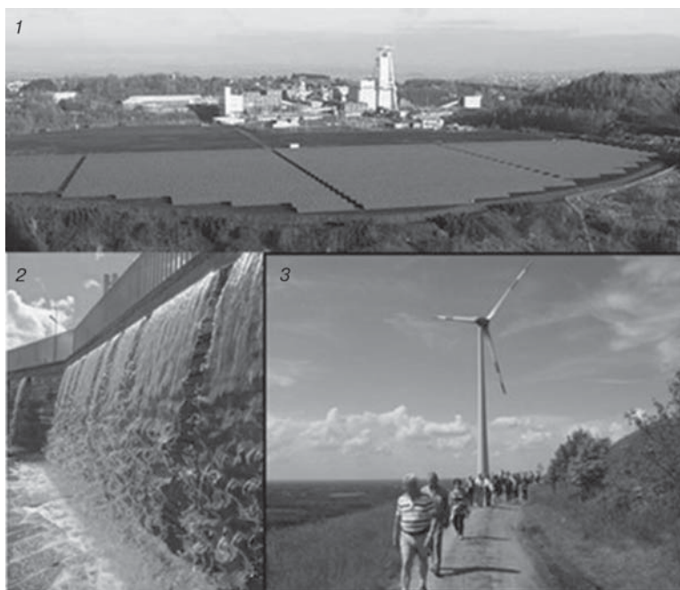
Fig. 3. Creating renewable energy, an opportunity of post-mining: 1 — Photovoltaic plant on a mud pond; 2 — Heat from mine water; 3 — Windmill on a dump hill
