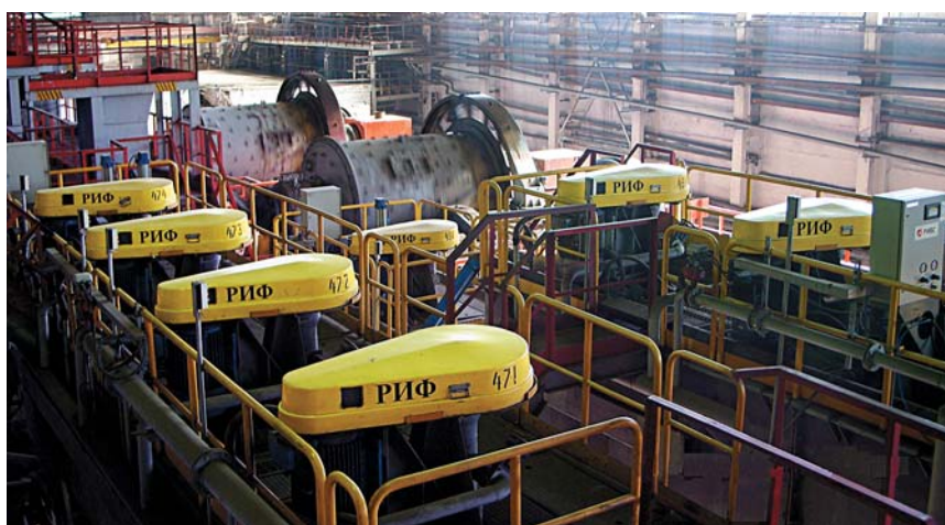
Fig. 8. Section of finishing of the rough zinc concentrate at Uchalinskaya concentrating plant
