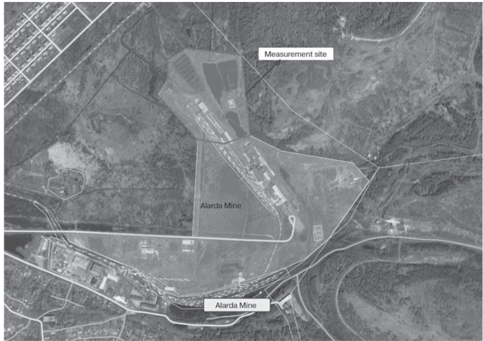
Alarda Mine field above the accident site of beds 1, 3 and 6 (scale 1:20000)
