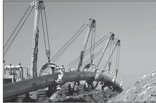
**Fig. 4. The pipes' bending of the main pipeline "Eastern Siberia – Pacific Ocean" under laying on the bottom of the trench**
