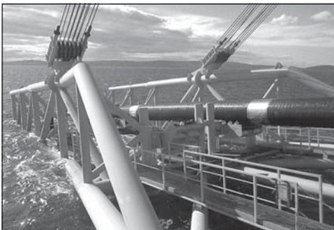
**Fig. 3. The laying of the main pipeline "Turkish stream" on the Black Sea bed by means of a stinger (S-lay method)**
