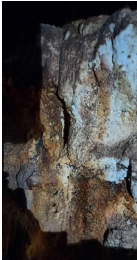
Fig. 6. Fracture in cast-iron tubing (level 88–89 in the shaft) and horizontal section at level 88 at elevation –145.275 m
