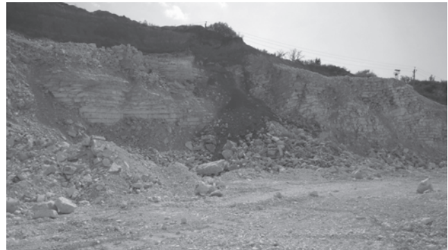
Fig. 4. Result of rotational landslide on pitwall slope
